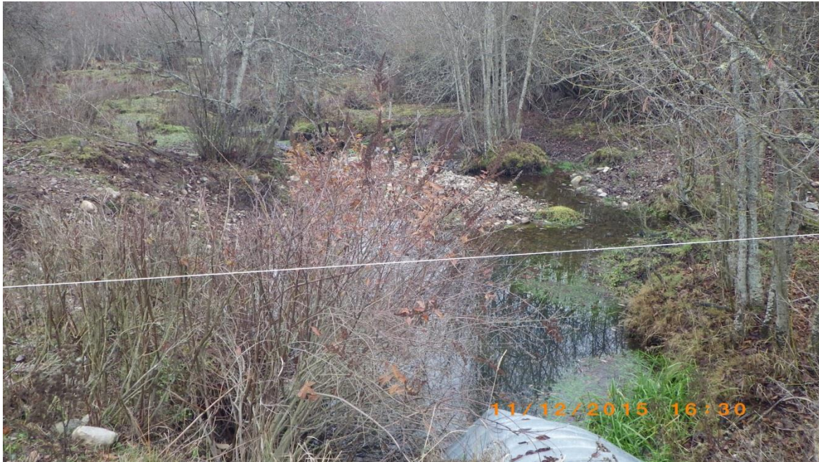
Figure 14. Erosion at outlet of upper Cocolalla Creek crossing.
