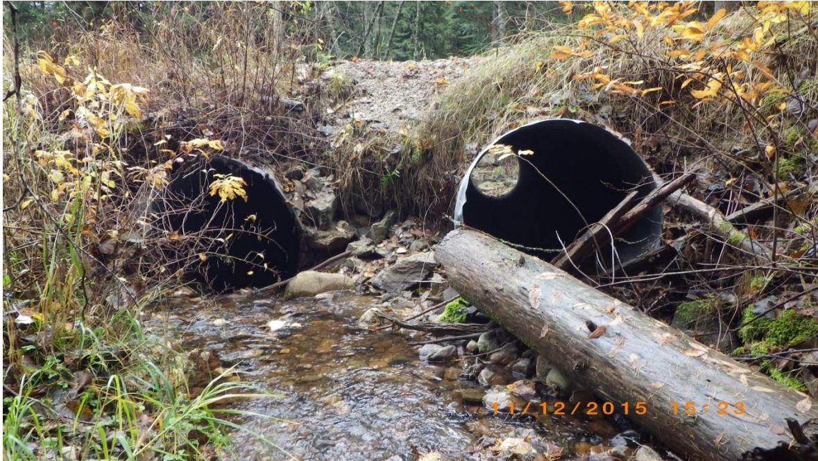
Figure 16. Road fill erosion into Fish Creek.
