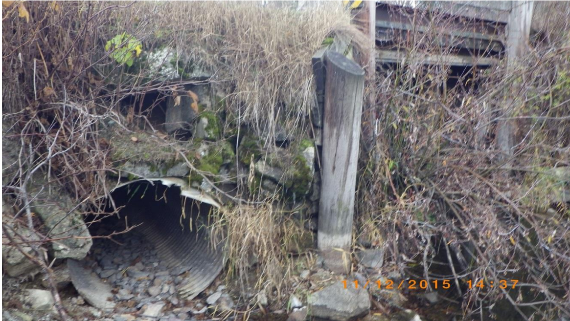
Figure 18. Rusted-out, overflow culvert at outlet of Cocolalla Lake.
