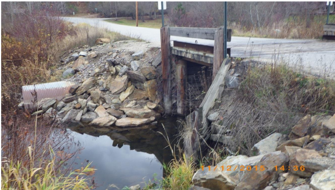
Figure 17. Undersized bridge at outlet of Cocolalla Lake.
