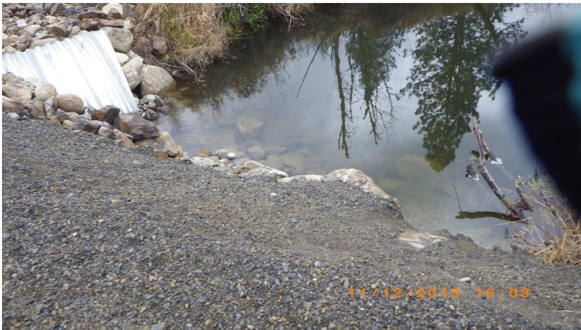
Figure 15. Road fill erosion into upper Cocolalla Creek.
